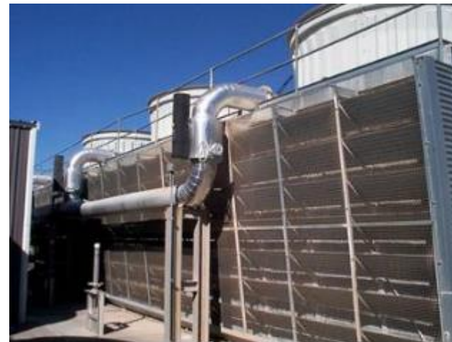
Cooling tower and HX = Water-side Economizer
