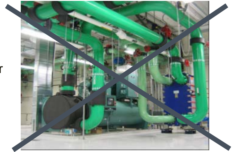
Cooling tower and HX = Water-side Economizer
